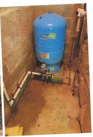
Pictures from left to right The well is located next to the road in front of the house. the well was installed 9/17/1991 which produces 5 gal/min 7200 gal/day. Depth of the well 405 ft deep with the casing 130 ft. The well is in working condition and will supply enough water for the home. Pressure tank is located in a closet facing the front of the house. Have any questions please give me a call.
