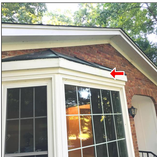
1.2 Item 3 No gutters
