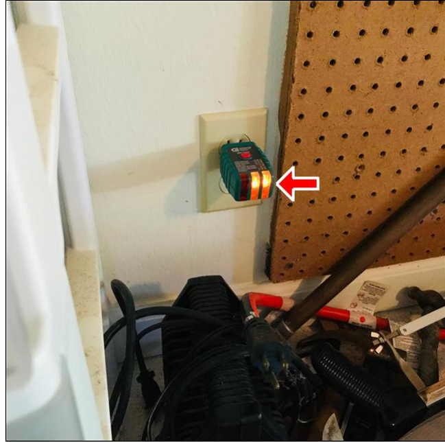
6.4 Item 2 No GFCI, garage
