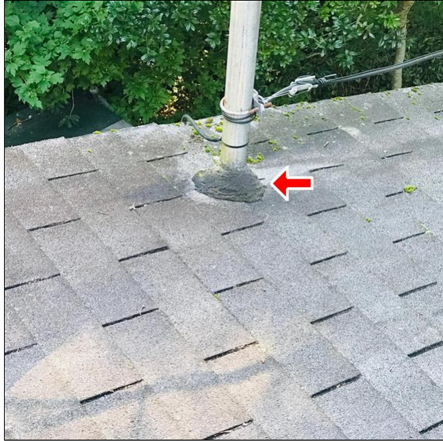
1.1 Item 2 Tared flashing
