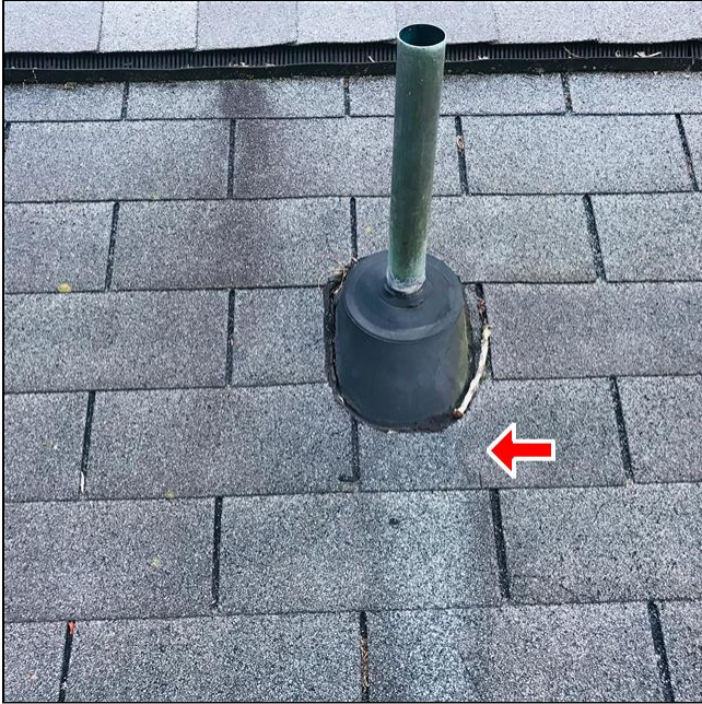
1.1 Item 1 Shingles over flashing
