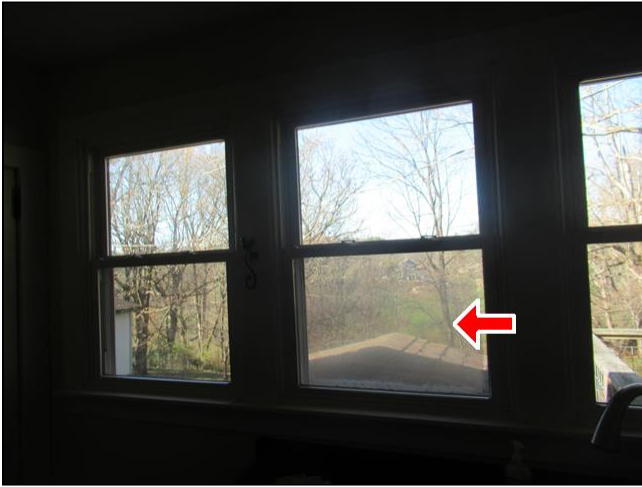
3.4 Item 1(Picture) kitchen window
