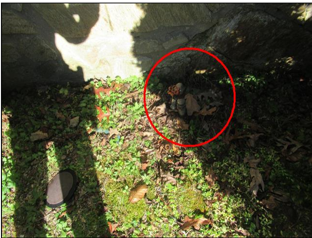
2.6 Item 1(Picture) galvanized plumbing
