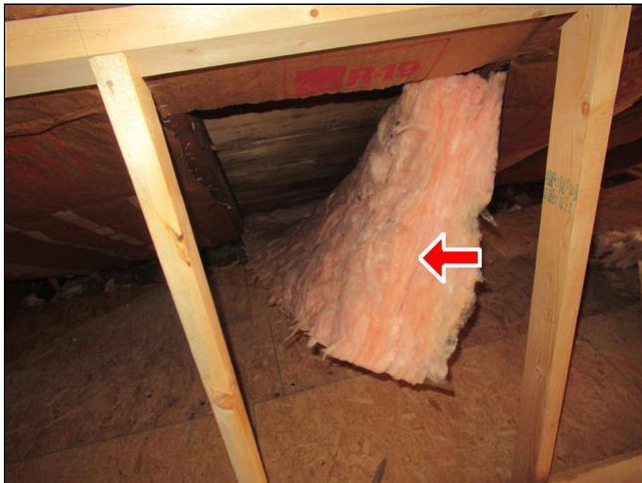
1.7 Item 3(Picture) secure the insulation
