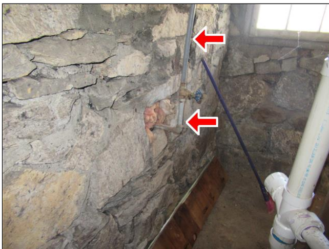
7.1 Item 1(Picture) galvanized and polybutylene
