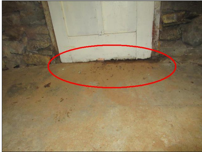
2.4 Item 2(Picture) basement door
