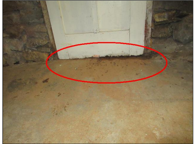
2.4 Item 2(Picture) basement door
