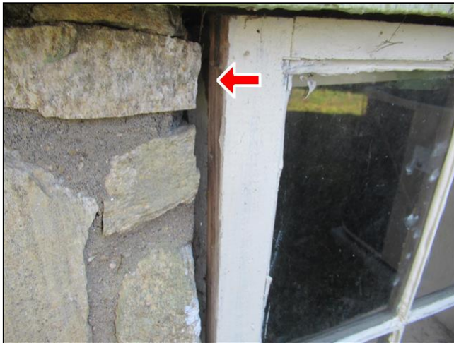
2.2 Item 1(Picture) right basement window
