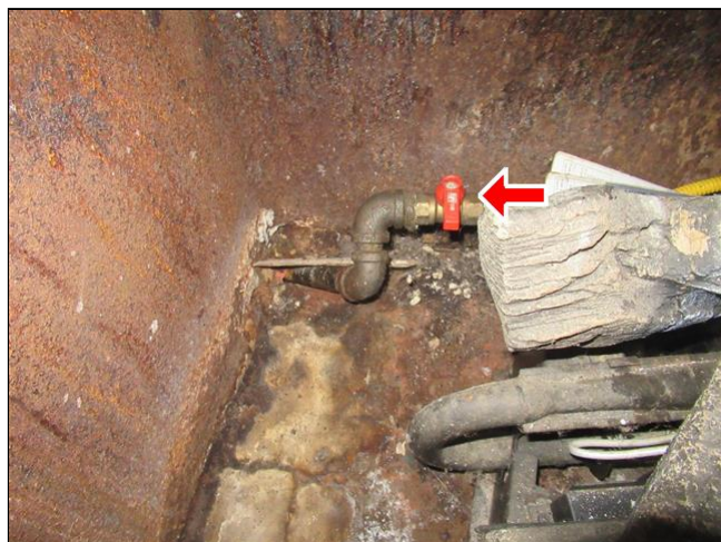
9.7 Item 1(Picture) gas shut off valve
