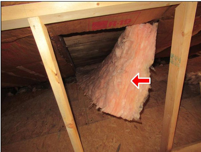
1.7 Item 3(Picture) secure the insulation
