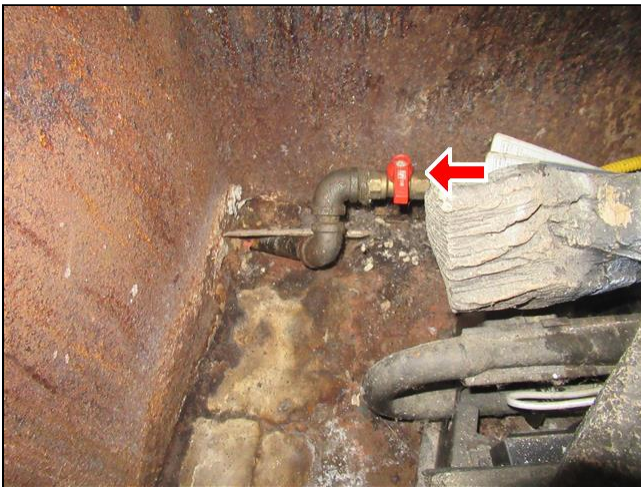
9.7 Item 1(Picture) gas shut off valve
