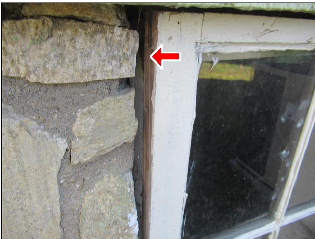
2.2 Item 1(Picture) right basement window
